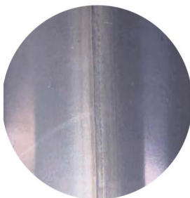
Welding can cause surface rusting.
